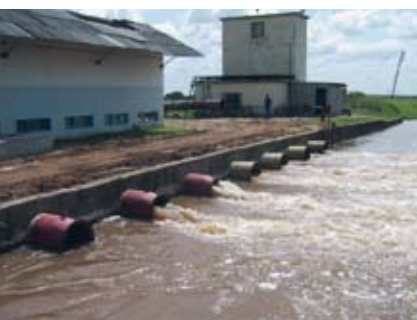
Return flow from Mafambisse sugar estate just upstream of Beira water intake, Mozambique. Photo: Björn Holgersson
