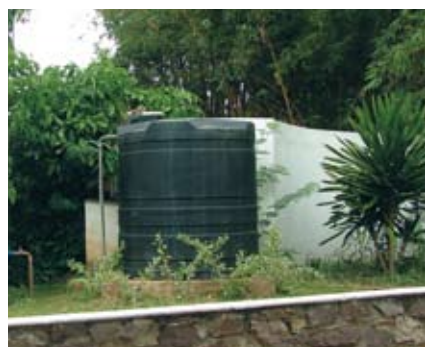
Water storage tank for household use in Maputo, Mozambique.
